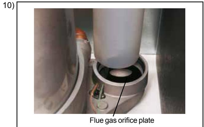
10) Place the flue gas orifice plate  $\varnothing$  53 mm into the condensate pan and insert the flue pipe again.
