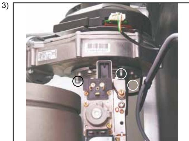
Unscrew the mixing chamber from the fan (three Allen screws 5 mm), and remove air inlet pipe if necessary
