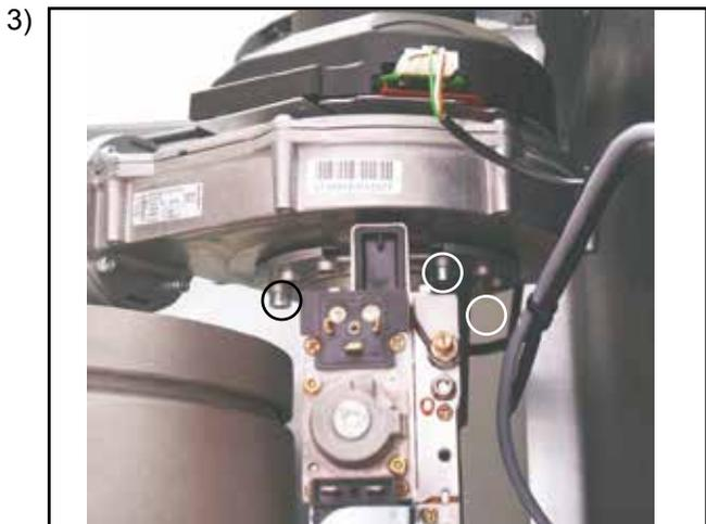
3) Unscrew the mixing chamber from the fan (three Allen screws 5 mm), and remove air inlet pipe if necessary
