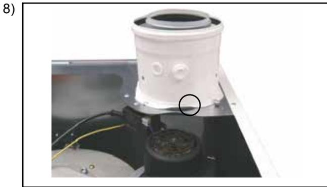
8) After removing the upper casing cover, undo the self-tapping screw at the balanced flue locking mechanism.
