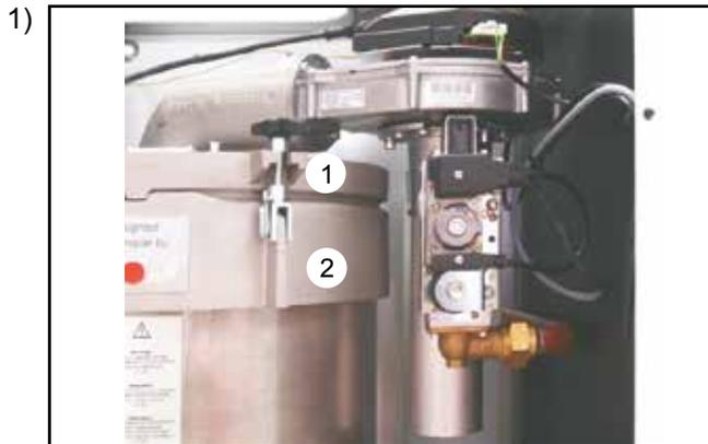
Unplug the connector ①② (first unscrew the Phillips head screws)
