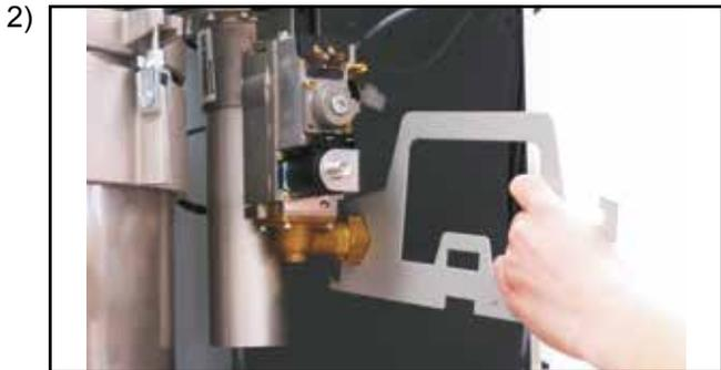
2) Undo gas connection at the gas combination valve
