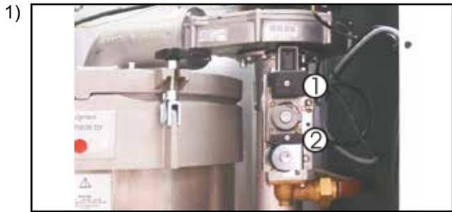
1) Unplug the connector ①② (first unscrew the Phillips head screws)
